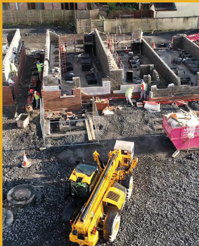
Site works at Mullingar, Co. Westmeath
