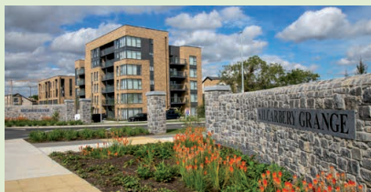
Kilcarbery Grange, Clondalkin, Co. Dublin
