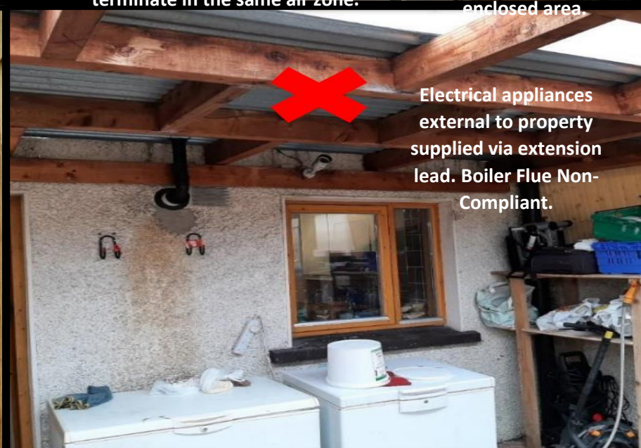
Air intake and exhaust must terminate in the same air zone.
